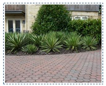
PERMEABLE SURFACES ARE SUITABLE FOR PEDESTRIAN AND/OR VEHICULAR TRAFFIC, WHILE ALLOWING RAINWATER TO INFILTRATE THROUGH THE SURFACE INTO UNDERLYING LAYERS
