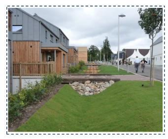
**SWALES** ARE SHALLOW, BROAD AND VEGETATED CHANNELS DESIGNED TO STORE AND/OR CONVEY RUN-OFF & REMOVE POLLUTANTS
