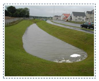
**DETENTION BASINS** PROVIDE A STORAGE FACILITY WITHOUT PERMANENT WATER & OFTEN HAVE A GRAVEL BASE TO ENSURE GOOD DRAIN DOWN. DETENTION BASINS TEND TO BE USED FOR LARGER DEVELOPMENTS
