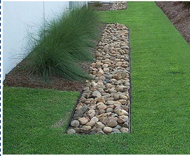
**INFILTRATION TRENCHES** ARE STONE-FILLED RESERVOIRS TO WHICH STORMWATER RUN-OFF IS DIRECTED, AND FROM WHICH THE WATER GRADUALLY INFILTRATES INTO THE GROUND
