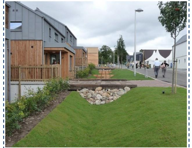
**SWALES** ARE SHALLOW, BROAD AND VEGETATED CHANNELS DESIGNED TO STORE AND/OR CONVEY RUN-OFF & REMOVE POLLUTANTS
