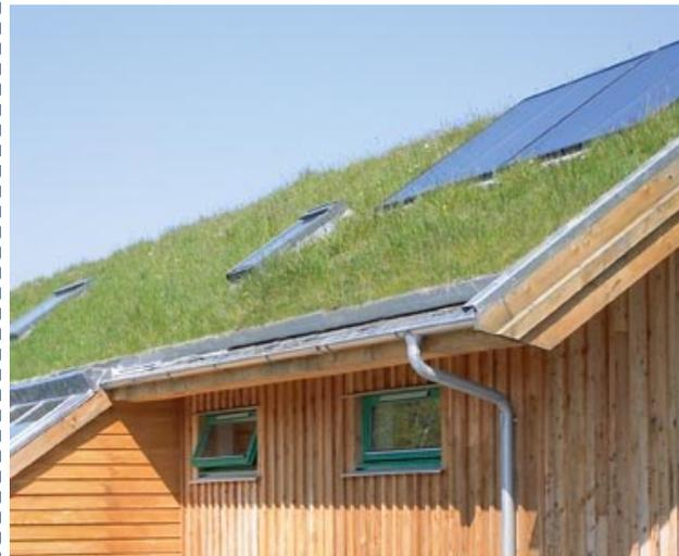
**GREEN ROOFS** ABSORB AND STORE RAINWATER AND FILTERING ANY POLLUTANTS. THEY ALSO PROVIDE HABITATS FOR WILDLIFE WHILST PROVIDING INSULATION
