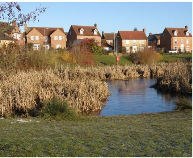
**RETENTION PONDS** PROVIDE BOTH STORMWATER ATTENUATION & TREATMENT. THEY PROVIDE PERMANENT WATER STORAGE & ARE DESIGNED TO SUPPORT AQUATIC VEGETATION ALONG THEIR SHORELINE
