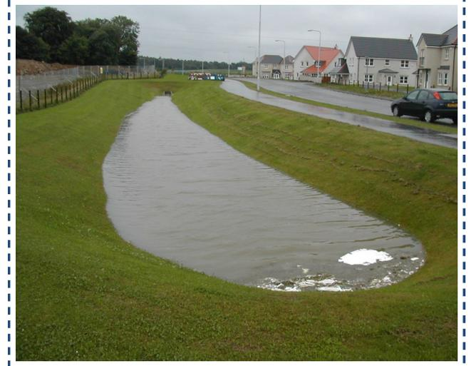
**DETENTION BASINS** PROVIDE A STORAGE FACILITY WITHOUT PERMANENT WATER & OFTEN HAVE A GRAVEL BASE TO ENSURE GOOD DRAIN DOWN. DETENTION BASINS TEND TO BE USED FOR LARGER DEVELOPMENTS
