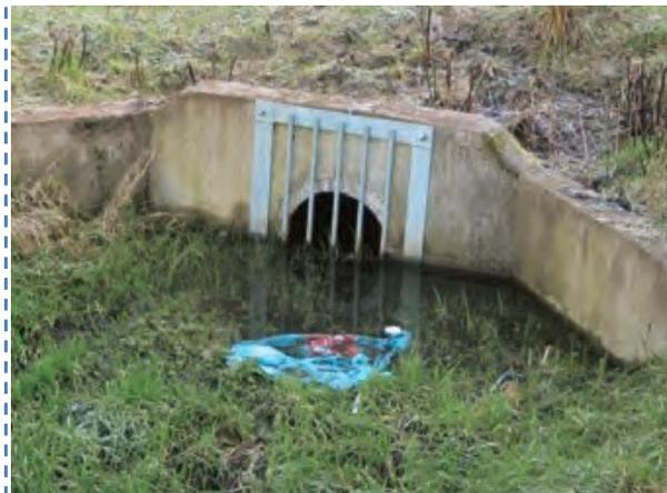
BLOCKED OR PARTIALLY BLOCKED INLET/OUTLET PIPES DUE TO A PROBLEM WITH DRAINING CAN RESULT IN FLOODING UPSTREAM AND POOR WATER QUALITY DUE TO STAGNANT WATER AND POOR SEDIMENTATION MANAGEMENT
