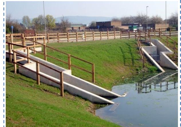
FENCING DETRACTS FROM THE AMENITY VALUE AND THE AESTHETIC QUALITY OF FEATURES, IT ALSO ACTS AS A BARRIER TO EFFICIENT MAINTENANCE. WELL DESIGNED SUDS SHOULD GENERALLY NOT REQUIRE FENCING
