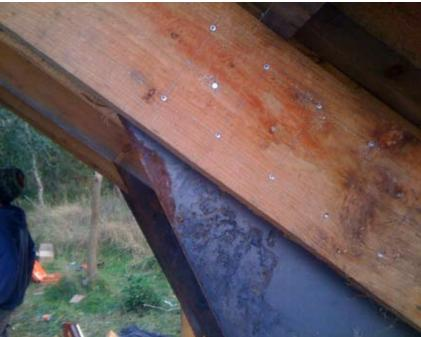
Fig. 21. Rafter-post connection detail prior to site application of metal paint
