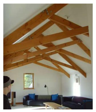
Fig.5. Timber/steel flitch beams with exposed bolts
