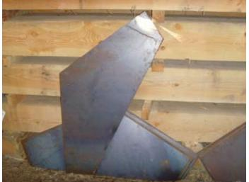
Fig. 19. Rafter to post steel connector plate
