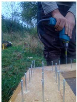
Fig. 20. Dowels being inserted on site with hand drill
