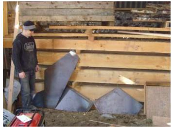
Fig. 18. Steel connection plates (left: rafter to post, right: ridge plates)
