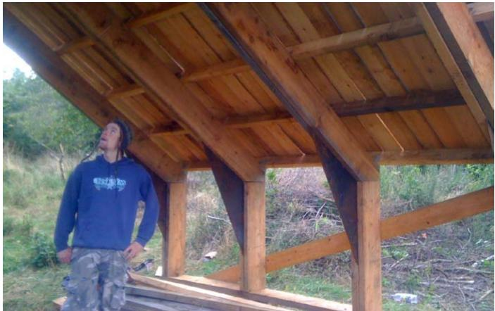
Fig. 22. Shelter constructed. Note construction of rafters with purlins on top, and vertical sarking boards. Also note barely-visible dowel connectors
