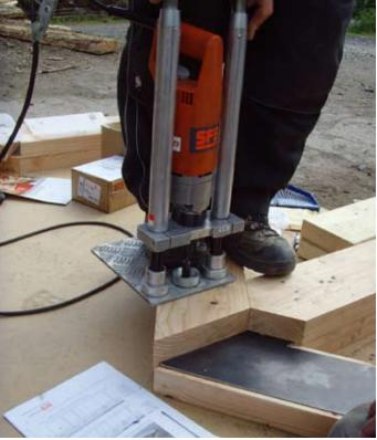
Fig. 13. Dowel inserted by driving down through timber and steel components
