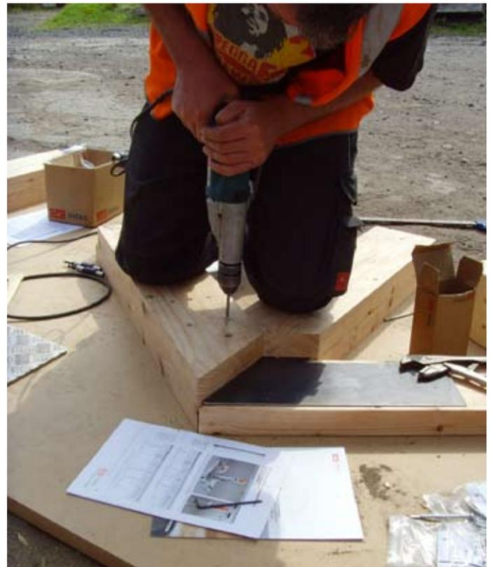
Fig. 15. Using hand drill to insert dowels, which achieved same effect.
