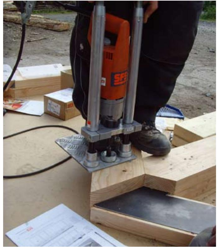
Fig. 13. Dowel inserted by driving down through timber and steel components
