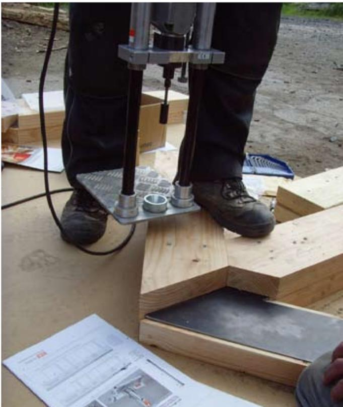
Fig. 14. Inspecting inserted dowel to ensure head is flush with timber surface
