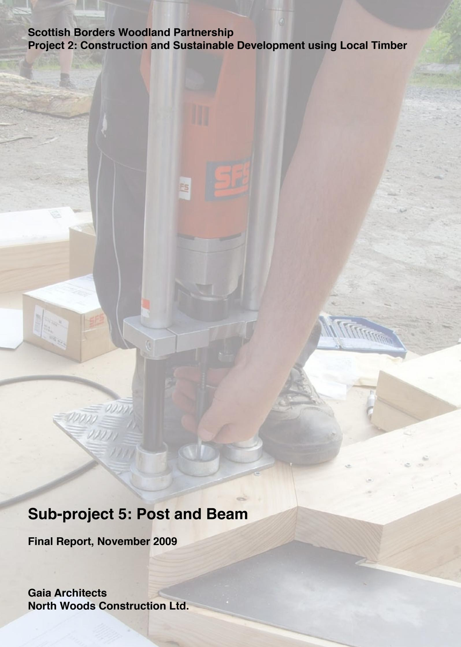
A person is using a hand-operated SFS post-hole drill to create a hole in a wooden beam. The drill is orange and silver, with the SFS logo visible. The person's hand is on the handle, and the drill bit is positioned in the wood. The background shows a construction site with wooden beams, a cardboard box, and a person's legs in the distance.
