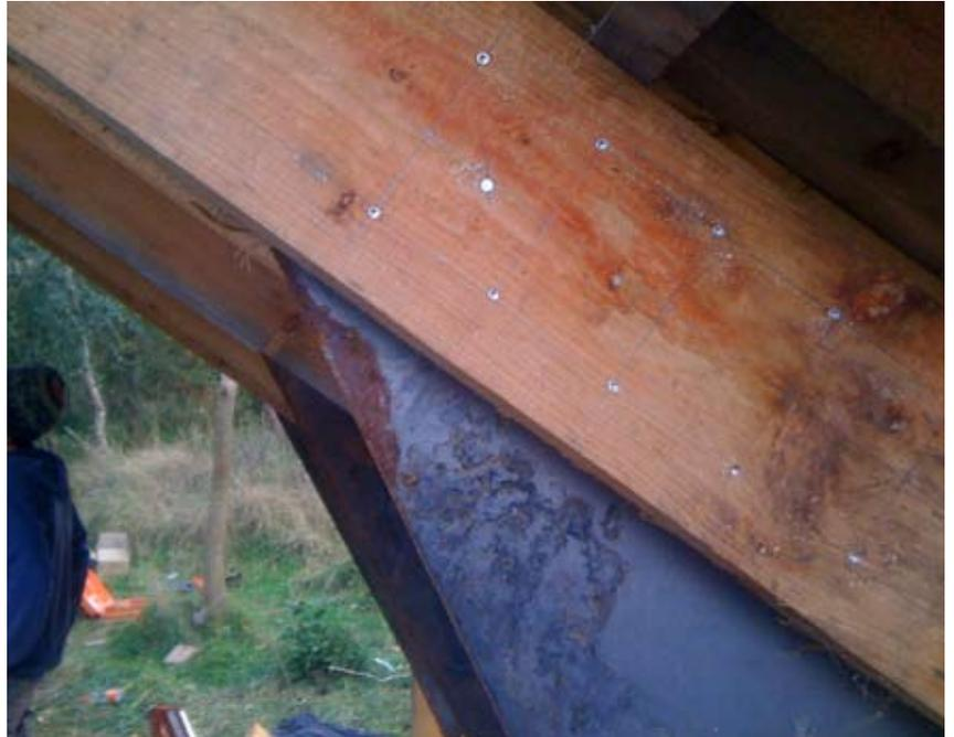
Fig. 21. Rafter-post connection detail prior to site application of metal paint
