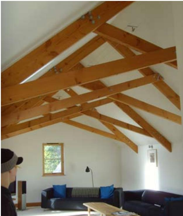
Fig.5. Timber/steel flitch beams with exposed bolts
