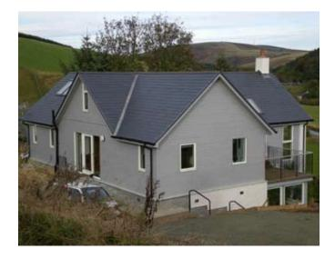
The house has 40 degree pitched, slated roof with a combination of coated cladding and rendered walls, with a grey brick base course. The gable facing east towards the A7 was changed from timber cladding to rendered blockwork during the design process, at the request of Scottish Borders Council Planning Department.
