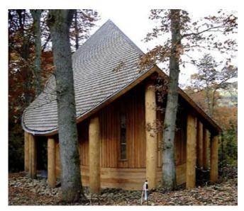
**Walls:** Upper part - vertical untreated Douglas Fir, square profile 250x25 and 200x25mm in board on board pattern on 25x47mm untreated battens and counterbattens. Lower part - 150x25mm horizontal Douglas Fir cladding with chamfered edges. All walls lined internally with v-jointed t&g softwood boards. All cladding stainless steel screw-fixed to battens.
