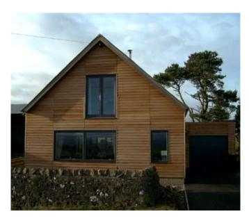
**Frame :** Roof, external walls & first floor structure in 350 & 300mm deep Masonite engineered I-joists; softwood framing for internal partitions.
