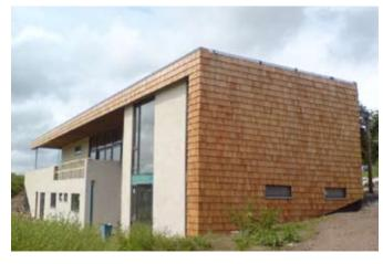
**Frame :** All timber framed: Parallam beams with masonite walls, floor & roof fully-filled with recycled newspaper insulation, built off a concrete slab foundation.
