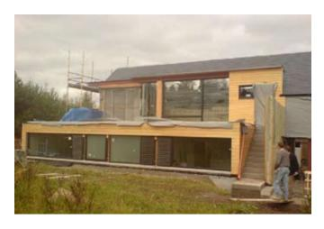
**Frame :** 225mm softwood framing in walls & roof, with steel frame around main stair and large glazed openings in Upper floor.
