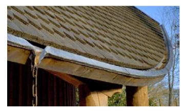
**Timber sources:** All timber used was grown and milled in Scotland. All Larch is heartwood of European Larch. The building has been detailed to ensure that timber is allowed to dry properly if it gets wet - this allows it to be used untreated.
