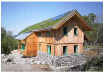
**Frame:** Highland Douglas fir 200x200mm posts, doubled 100x350mm beams to Post & Beam frame. Wall Panel and purlin framing in 44x197 regularised C16 Highland Spruce.
