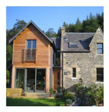
**Details:** Windows are FCS redwood. Oak window sills, with sub-frames and facings in Douglas Fir. Internal door reveals in oak. Front door is Douglas Fir stiles and rails with Siberian Larch infill panels.
