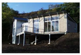
**Frame :** A hybrid post and beam frame with stud framed exterior walls. 200mm softwood framing in walls; 250mm in roof. The elevated ground floor area and adjoining deck is on a steel sub-base.
