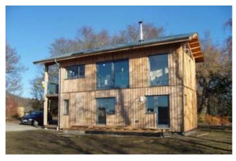
**Frame:** The entire structure with the exception of the large section exposed Douglas and Larch elements was resourced in 220x44 C16 regularised Spruce supplied by James Jones. This was an intentional simplification and design response to the material rather than the material responding to the design intention.
