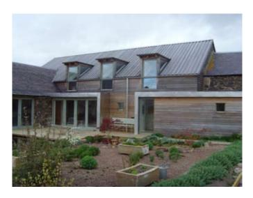
**Cladding:** 150 x 20mm Siberian larch shiplap boarding with plane angled exposed surface, stainless steel nailed to counter-battens. Stainless steel cladding to link corridor.
