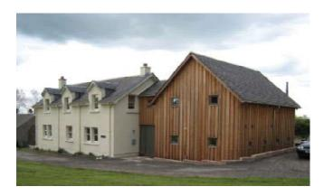
**Cladding:** 150 x 20mm Siberian larch set board-onboard, stainless steel nailed to counterbattens.
