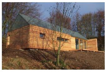
**Timber sources:** The timber frames are untreated Scottish softwood in prefabricated panels supplied by ARM Buildings. Douglas fir beams and European larch supplied by local sawmill, Abbey Timber. Scots Pine glulam post and beam supplied by Norbuild of Forres. Redwood windows and external doors from various sources.
