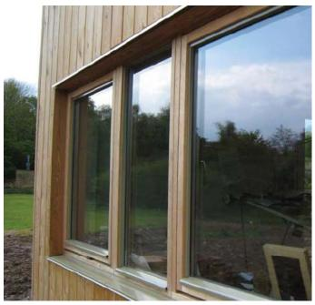
Difficulties & constraints: Architect favoured use of local home-grown larch for cladding but, along with client, felt that what was available locally was unsuitably – preponderance of knots and varying grain patterns made dressing very difficult and compromised weathering ability, particularly as cladding to be left unpainted/unstained to weather naturally. Some problems also with movement in softwood framing and decking, but this now resolved by
