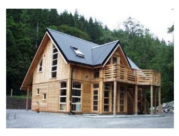
**Frame :** Post and beam spine in Douglas fir with pre-fabricated, pre-insulated panel construction. 200mm softwood framing in walls; 225mm in roof and exposed Douglas fir joists to first floor.
