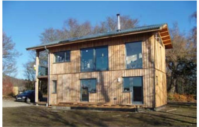
**Frame:** The entire structure with the exception of the large section exposed Douglas and Larch elements was resourced in 220x44 C16 regularised Spruce supplied by James Jones. This was an intentional simplification and design response to the material rather than the material responding to the design intention.
