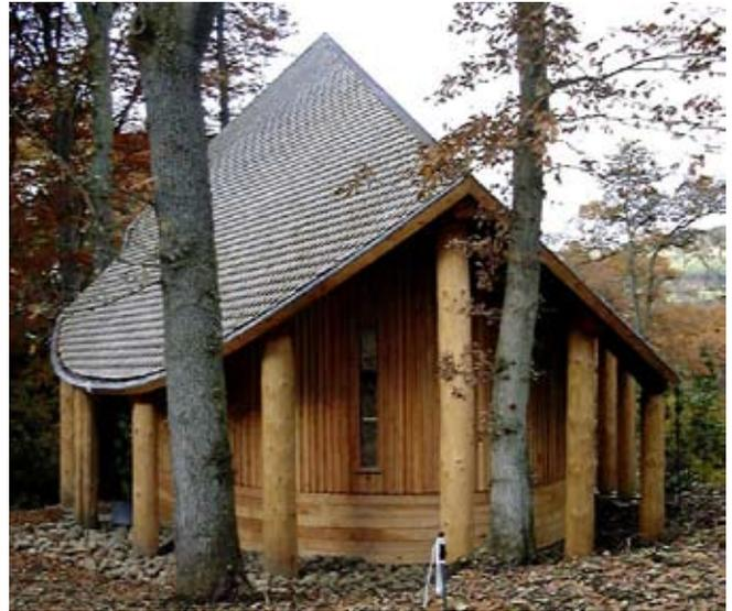
**Walls**: Upper part - vertical untreated Douglas Fir, square profile 250x25 and 200x25mm in board on board pattern on 25x47mm untreated battens and counterbattens. Lower part - 150x25mm horizontal Douglas Fir cladding with chamfered edges. All walls lined internally with v-jointed t&g softwood boards. All cladding stainless steel screw-fixed to battens.
