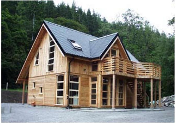
**Frame** : Post and beam spine in Douglas fir with pre-fabricated, pre-insulated panel construction. 200mm softwood framing in walls ; 225mm in roof and exposed Douglas fir joists to first floor.
