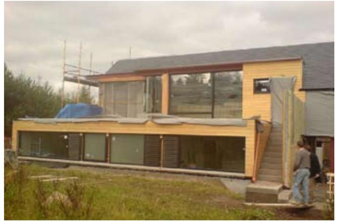
**Frame :** 225mm softwood framing in walls & roof, with steel frame around main stair and large glazed openings in Upper floor.
