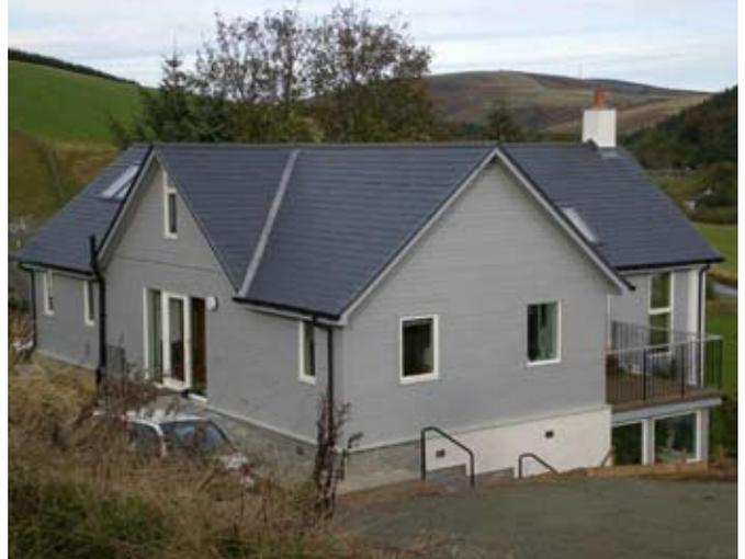
The house has 40 degree pitched, slated roof with a combination of coated cladding and rendered walls, with a grey brick base course. The gable facing east towards the A7 was changed from timber cladding to rendered blockwork during the design process, at the request of Scottish Borders Council Planning Department.
