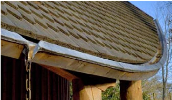
**Timber sources** : All timber used was grown and milled in Scotland. All Larch is heartwood of European Larch. The building has been detailed to ensure that timber is allowed to dry properly if it gets wet - this allows it to be used untreated.
