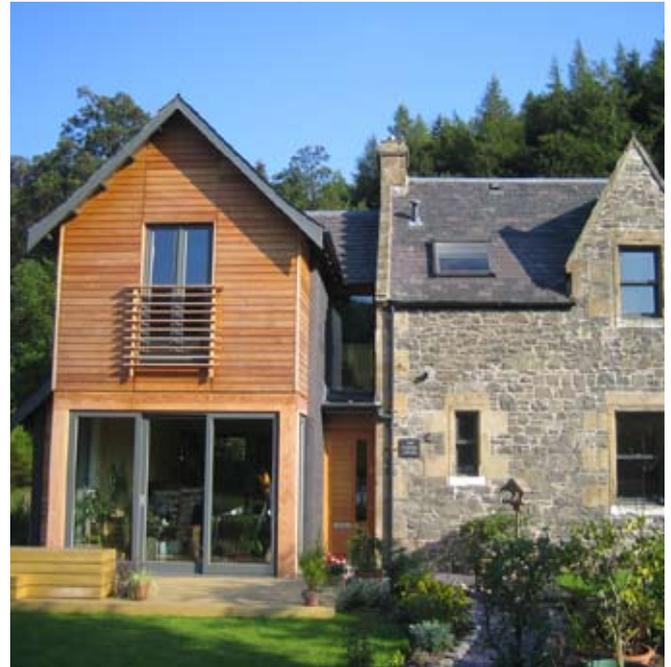
**Details** : Windows are FCS redwood. Oak window sills, with sub-frames and facings in Douglas Fir. Internal door reveals in oak. Front door is Douglas Fir stiles and rails with Siberian Larch infill panels.
