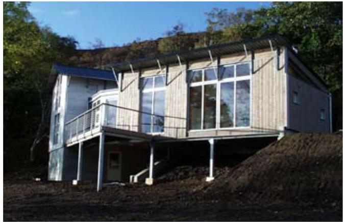
**Frame** : A hybrid post and beam frame with stud framed exterior walls. 200mm softwood framing in walls ; 250mm in roof. The elevated ground floor area and adjoining deck is on a steel sub-base.
