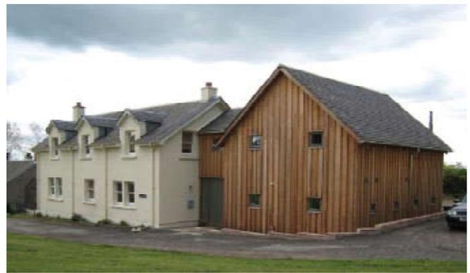
**Cladding** : 150 x 20mm Siberian larch set board-on-board, stainless steel nailed to counter-battens.
