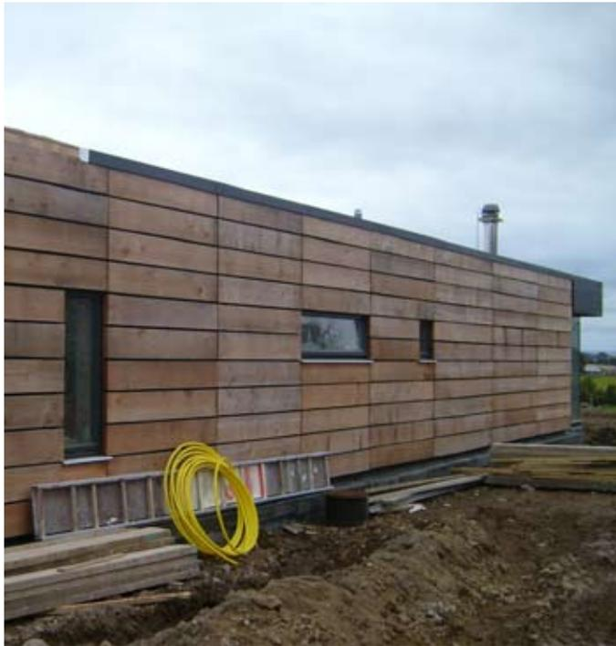
**Difficulties & constraints :** House half cut into site with the entrance at upper floor level, meant the non-timber elements (retaining wall & tanking)) were the most complicated to build. Once this was complete, the main frame & form of the building was relatively straightforward, with detailing & junctions the only real issues.
