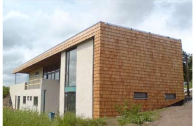
**Frame :** All timber framed: Parallam beams with masonite walls, floor & roof fully-filled with recycled newspaper insulation, built off a concrete slab foundation.
