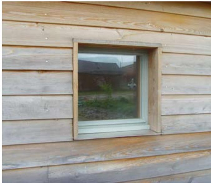
**Cladding** : 150 x 20mm Siberian larch shiplap boarding with plane angled exposed surface, stainless steel nailed to counter-battens. Stainless steel cladding to link corridor.
