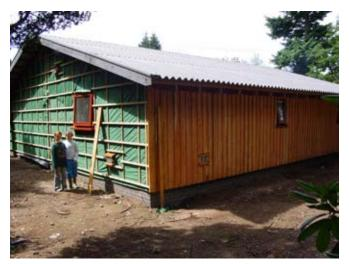
Figure 8. untreated, board-on-board vertical cladding
