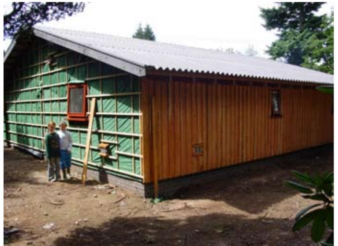
Figure 8. untreated, board-on-board vertical cladding
