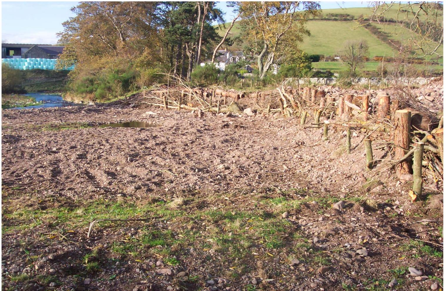
**Cheviot Futures 2.** Innovative bank Protection works. Protecting key infrastructure. Engineered Log Jam based on MNV suggested design.
