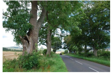
Ageing, potentially dangerous roadside trees
