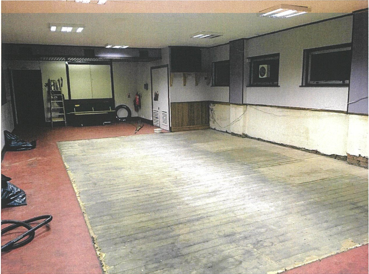
Ex Service Men's Club bar stripped out ready for Men's Shed to move in.
