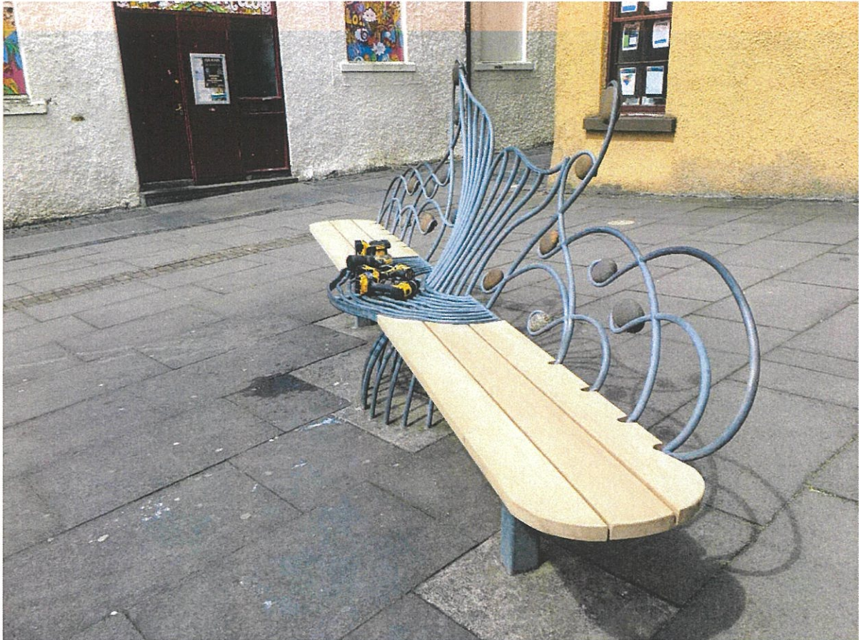
Ornamental bench on School Brae refurbished by cutting and fitting new oak slats.
