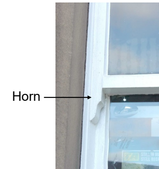
Figure 17: Traditional Window Detail - Horn Detail
