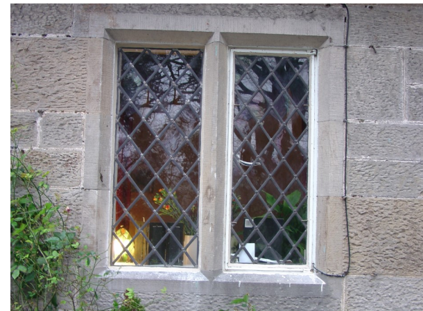
Figure 15: Traditional Metal Window with Lead Detailing on a Residential Property
