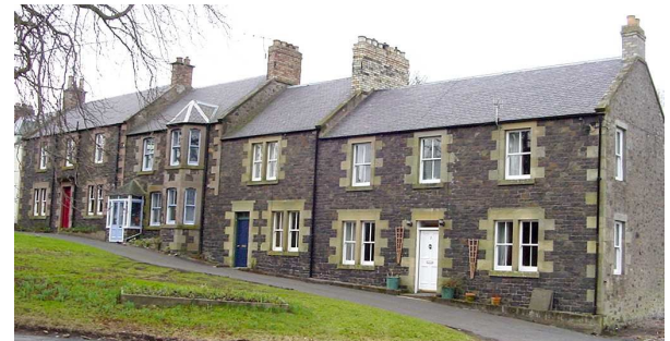
Figure 2: Historic Street Frontage - Yetholm
