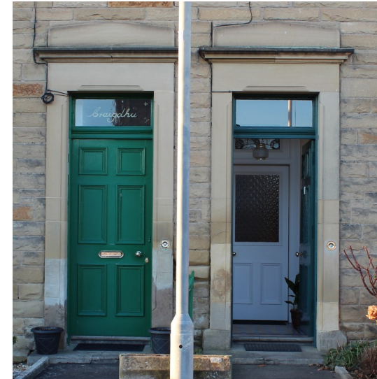
Figure 28: Matching Traditional External Doors (with internal door in entrance) - retaining matching doors on a street assists in protecting the character and appearance of the street.
