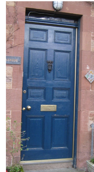
Figure 23: Example of a Panelled Main Entrance Door
