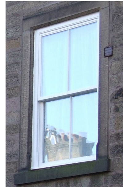
Figure 21: Acceptable Replacement Window
